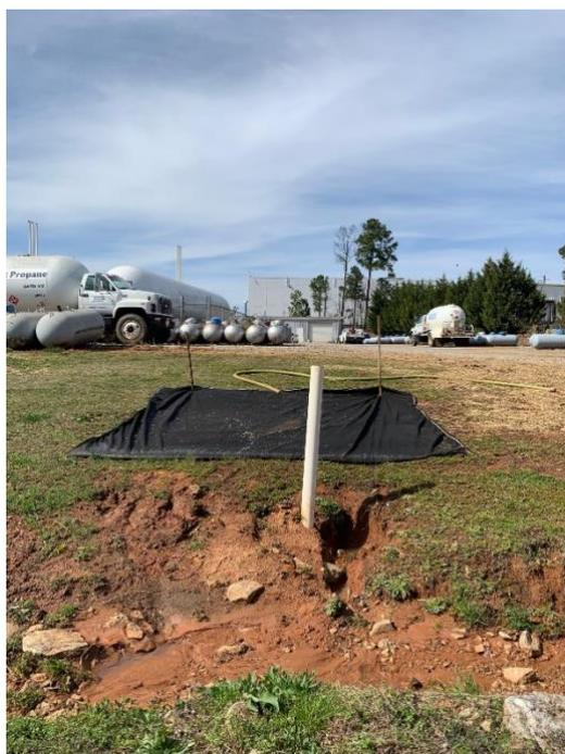
**Step 1:** Prepare your dewatering bag by lying it flat on the designated dewatering area. Dewatering bags can be placed in many different locations, but placing the bags on porous surfaces can help improve the overall performance of the dewatering bag. Bags may also be placed in dump trucks, dumpsters, or smaller container bins for storage and disposal purposes.
